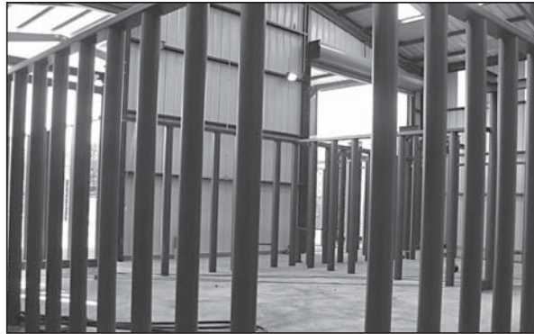
Heavy steel sections were included in the design to contain Gypsy the elephant in the facility. Photo by Cathy Burkey
